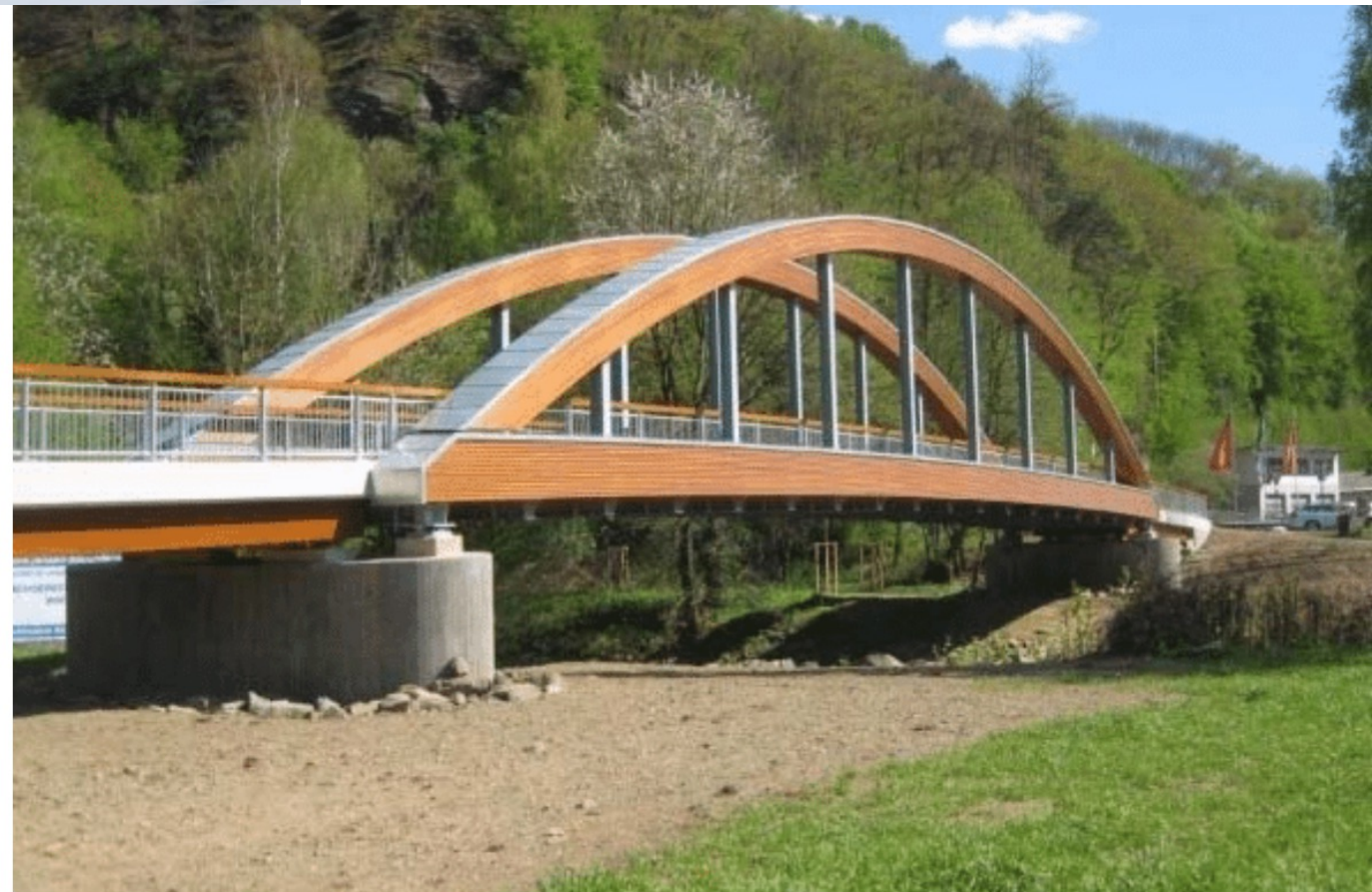
Timber bridge in Höngesberg (North-RhineWestphalia, Germany)
